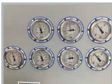
refrigerant and oil gauges
